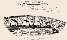
The bridge in the 17th century
